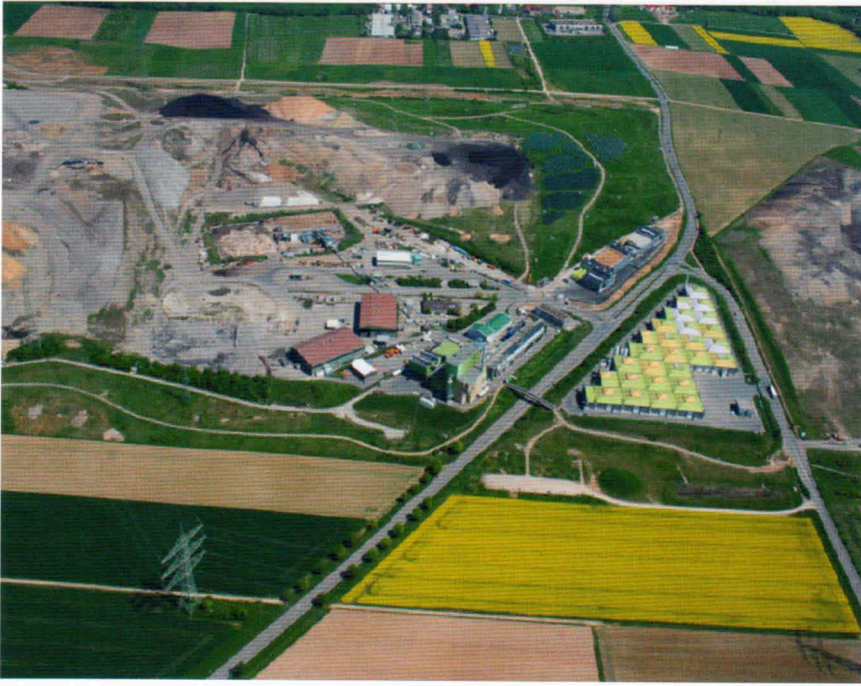
Figure 2: Aerial view of Rhein-Main Deponiepark in Flörsheim-Wicker
